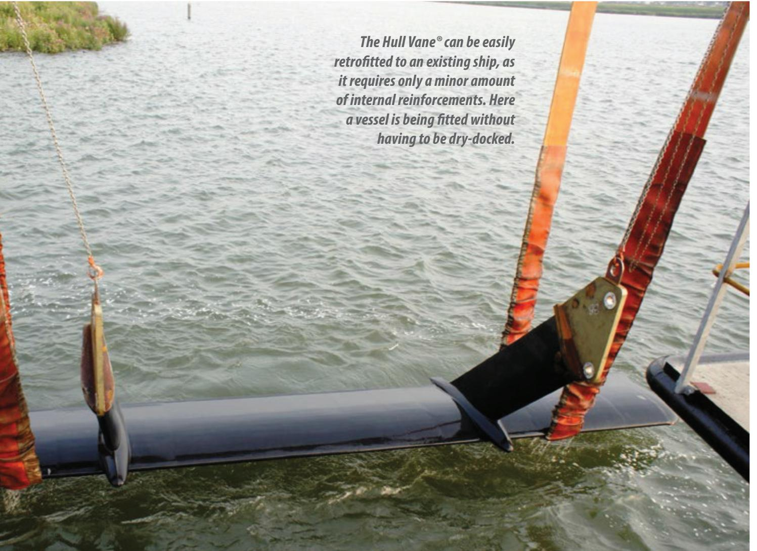
*The Hull Vane® can be easily retrofitted to an existing ship, as it requires only a minor amount of internal reinforcements. Here a vessel is being fitted without having to be dry-docked.*
