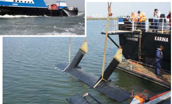
► From top: design image of the installed hull vane; MV Karina ; lifting the hull vane into position
